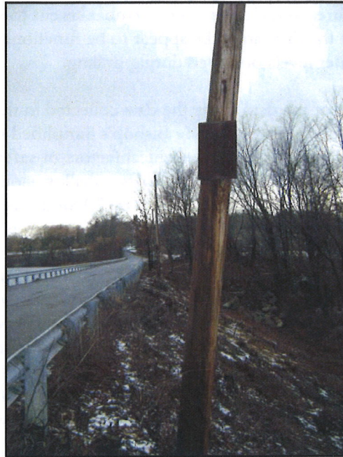
Note old rusted sign – plumb and level and guard rail – plumb and straight
